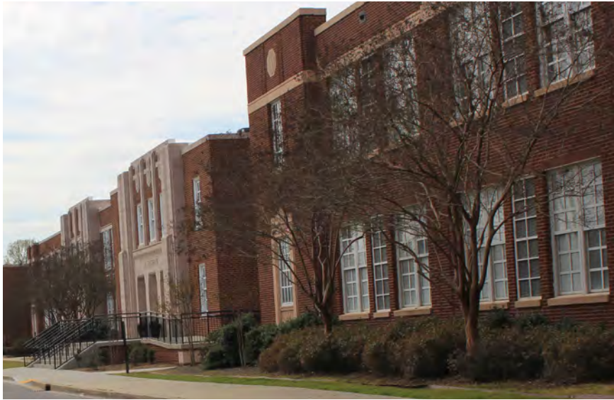
Auditorium entrance at Brookland Cayce High School.
