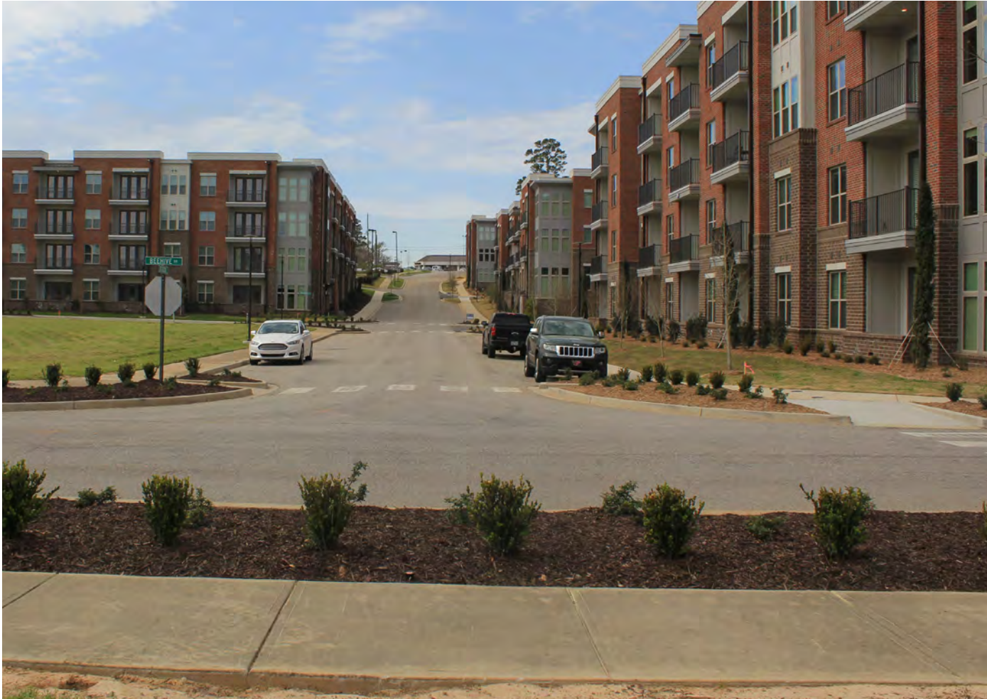
1. New multi-family housing being built in Cayce near the Congaree River. The development includes sidewalks and connectivity to commercial areas and the Three Rivers Greenway.
